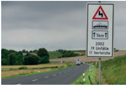
Before: poor marking – accident hot spot
