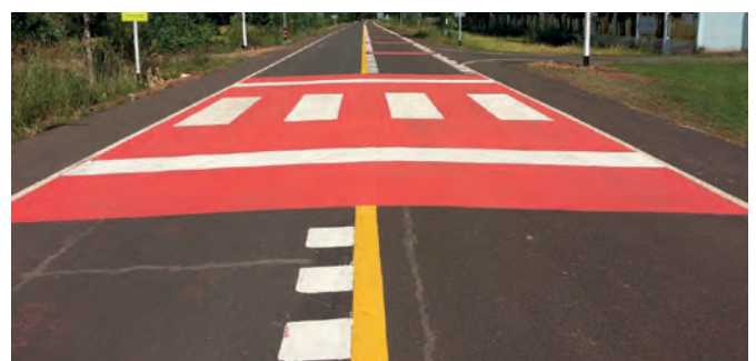
Photos © Department of Rural Roads, Thailand. Bureau of Traffic Safety
