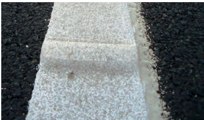
Form stable profile marking based on DEGAROUTE® based cold plastic MMA
